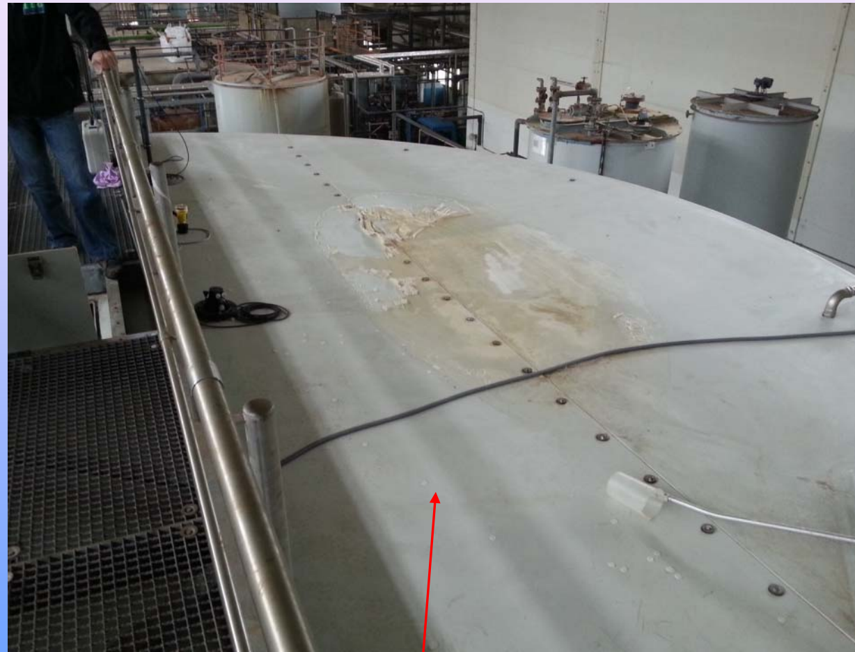
MBBR tank with cover, operated with Mutag BioChip™ carriers
